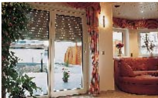
The blinds open and close dependent on time and external light
