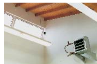
When the sky lights are opened, the fan heaters are automatically switched off during warm periods
