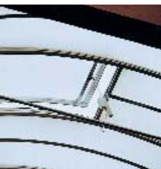
The control of shutters, fanlights and toilet windows is carried out via the bus
